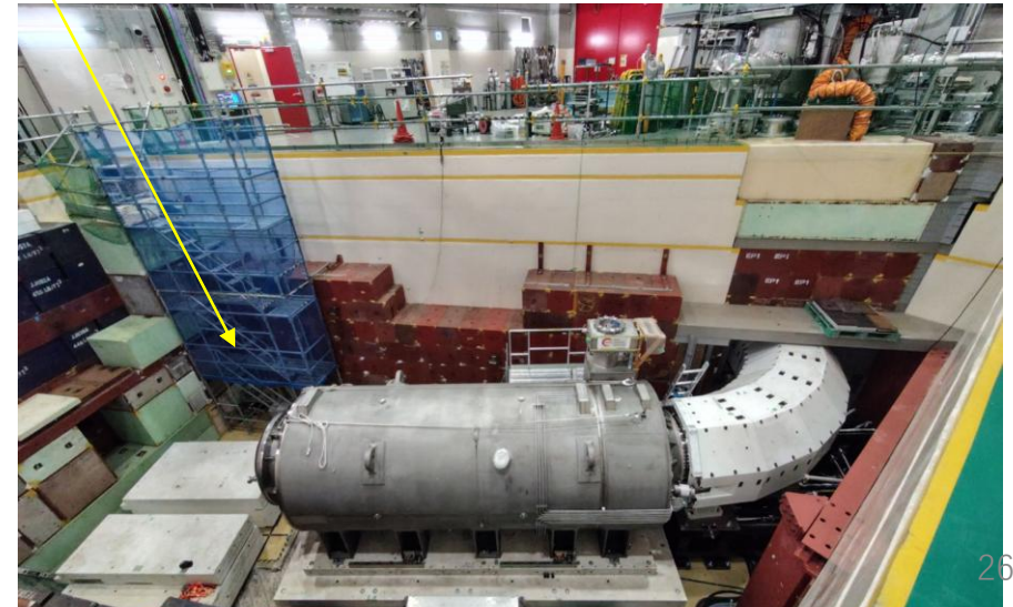
CS delivered and installed in Nov. 2024!
