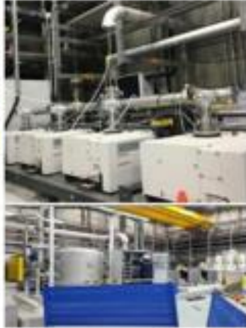
Compressors and Oil Removal System (WCS)
