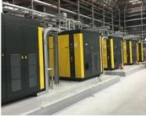
Compressors and Oil Removal System (WCS)
