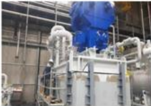
Compressors and Oil Removal System (WCS)
